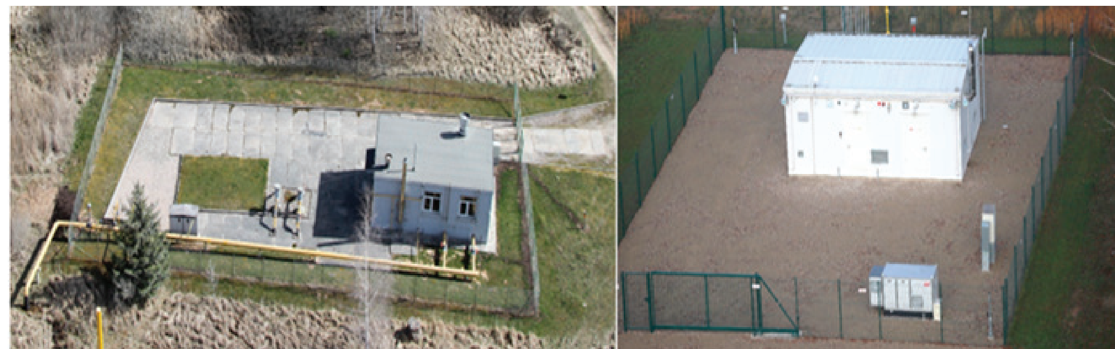
Figure 5.1. Gas regulation station Brocēni before and after reconstruction
